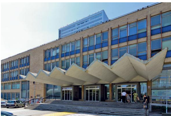
Main entrance (Image source: www.asb.sk )
