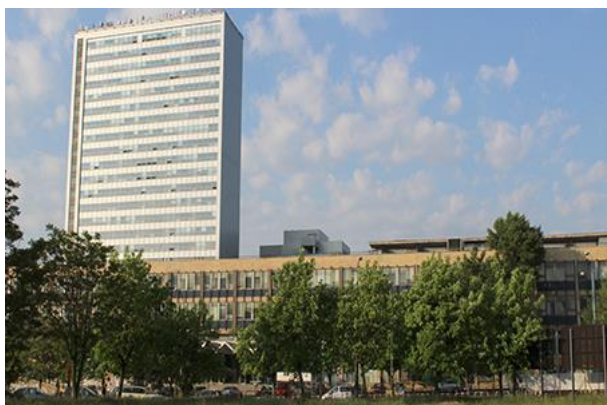
Building C (Image source: www.svf.stuba.sk )
